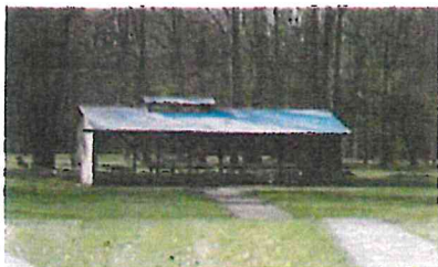
Wench Park - pavilion (no electricity) and restroom building - capacity 30-50
